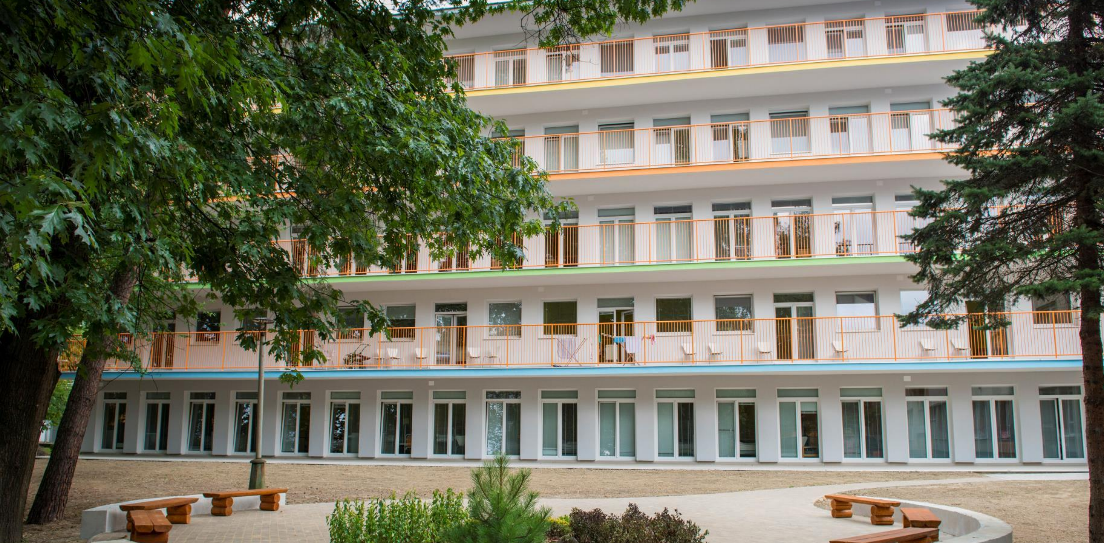
Zilina Faculty Hospital reconstruction (2014-2017)
